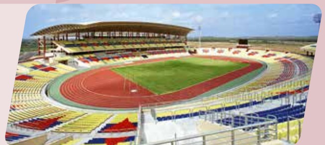
Hang Jebat Stadium, Melaka/Malaysia (MX system family)
